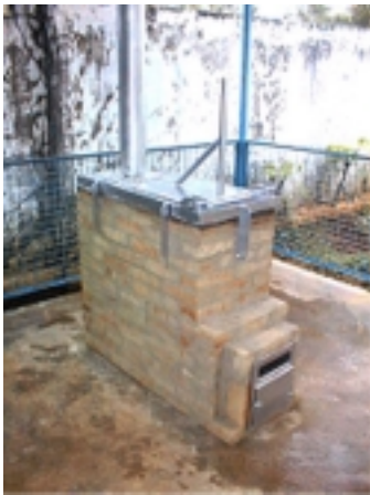
De Montfort small-scale incinerator, 600°-800°C
