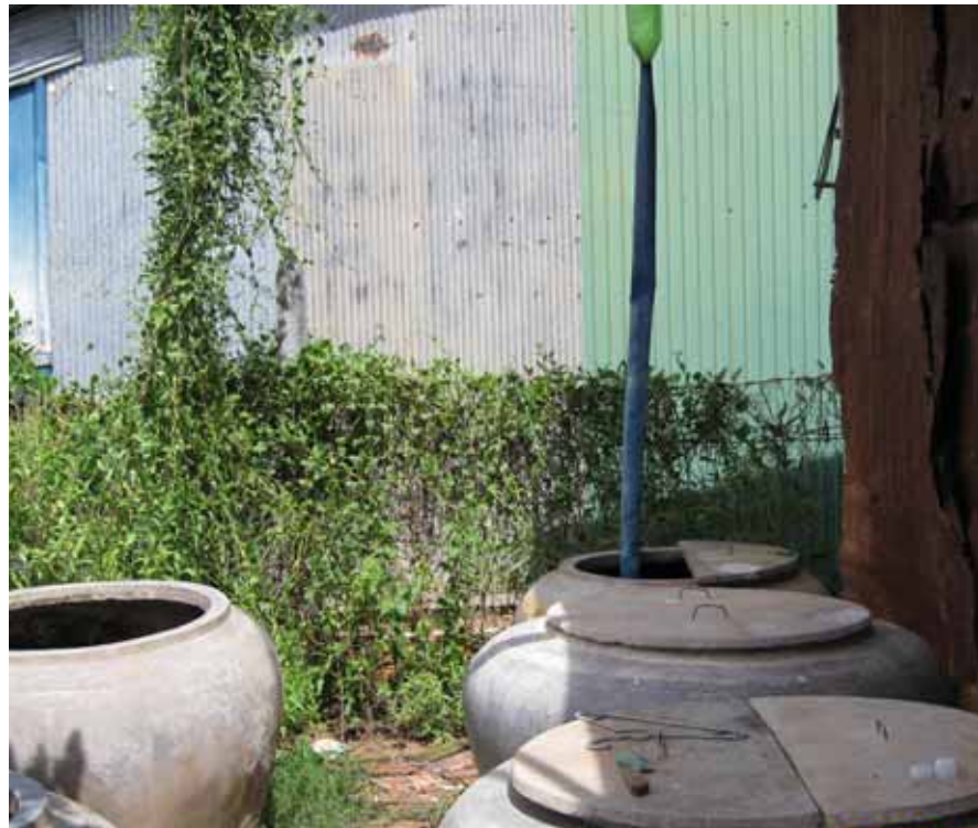
In the wet season, most Cambodians collect rainwater to drink because it is convenient, clean, and inexpensive. These large concrete jars are the most common way to store water in the home.
